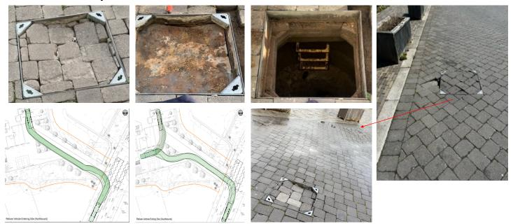
A number of defect have been raised regarding failures of recessed manhole covers, especially in vehicle trafficked paved areas, even though they are the correct heavy duty type:
