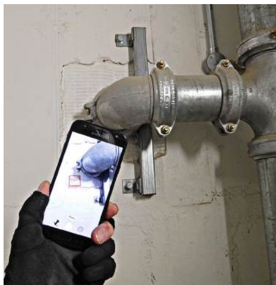
Figure 33 Electronic recording of a penetration seal installation
