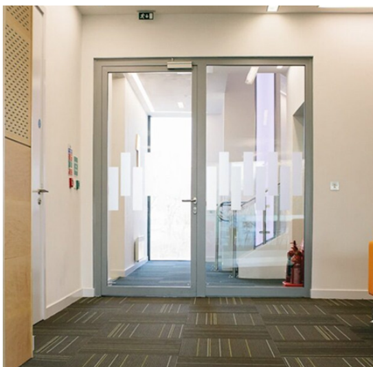
Figure 9 Fire resistant glazed side light and door in a supporting construction
