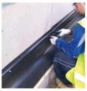
The increased use of SFS framing with sheathing board does not provide a mortar joint in which to bed the upstand of the tray and a detail must be provided on how the tray is secured to the sheathing board. The fixing specification, stainless steel, plastic etc. is important for corrosion, both from the environment and bi-metallic, and what the fixing is puncturing and providing a possible water ingress path. **Breather membranes should be dressed over the tray.**
